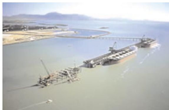
Courtesy of Major Metals Queensland Gladstone—RG Tanna Coal Loading Wharf
